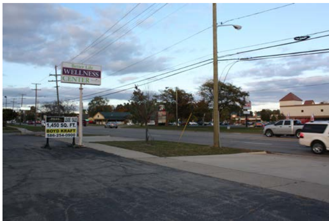
Van Dyke currently has a variety of frontages, small lots mixed with larger lots, unsightly parking and signage
