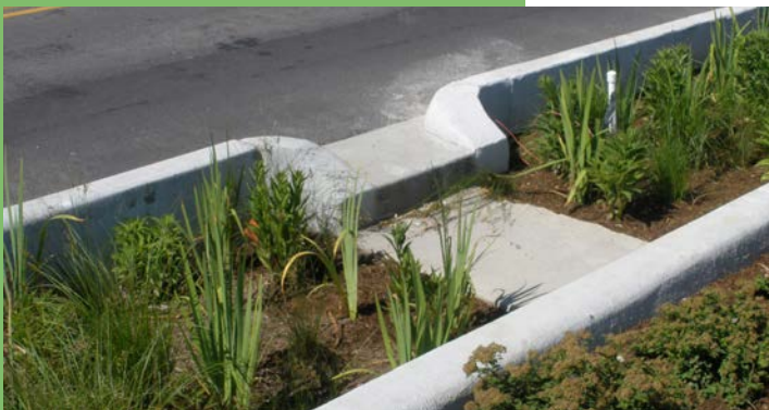
Example of bioswales treating runoff
