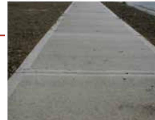
Picture frame border with brushed concrete finish
