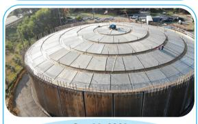
Oct. 11, 2021 Roof panels are put in place, enclosing the 3.5 million-gallon water storage tank.
