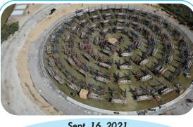
Sept. 16, 2021 Contractors install the flooring structure for the 3.5 million-gallon storage tank.
