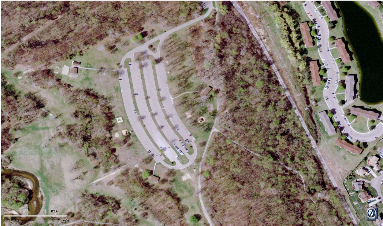
River Bends Park – 22 Mile Road Site
